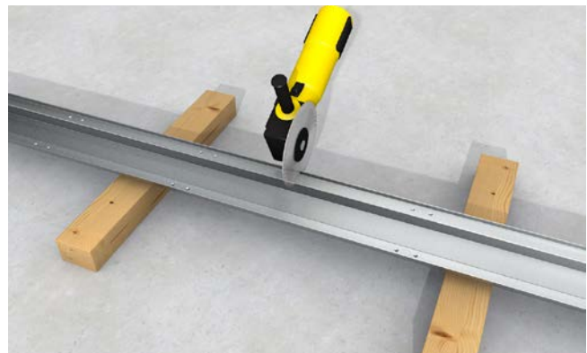
Cut the trunking segments and cover to size and check the fit in the milling zone.
